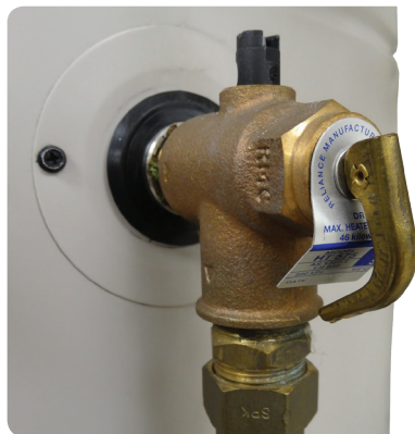
TPR position - top of cylinder
